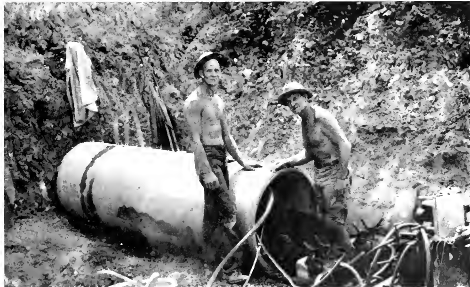
View of equipment and two-man crew used in jacking operations
